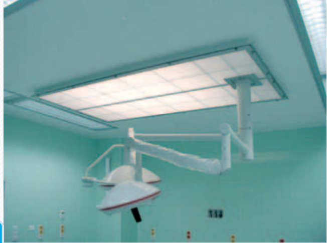
CG inlet ceiling - operating room in department of gynaecology
