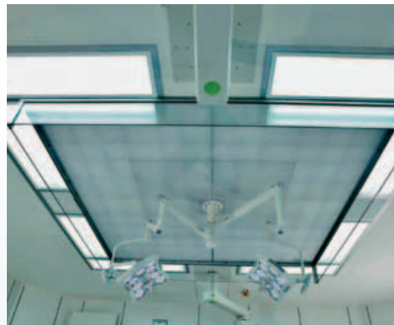
CG inlet ceiling
