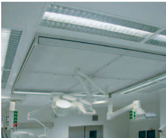
CG inlet ceiling
